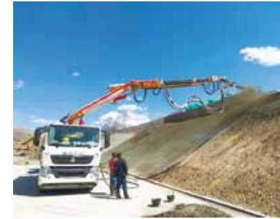
HPC30V混凝土喷浆车 张家口崇礼铁路太子城隧道 HPC30V truck-mounted concrete spraying machine Taizheng tunnel along Chongli railway in Zhangjiakou
