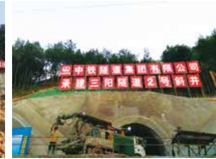
HPC30V混凝土喷浆车 福建三明兴泉铁路三阳隧道 HPC30V truck-mounted concrete spraying machine Sanyang tunnel along Xingquan railway in Sanming, Fujian
